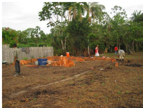
Anori – raising the walls
