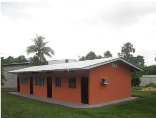
New roof on Institute classrooms
