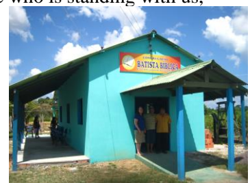
New work on KM 6
