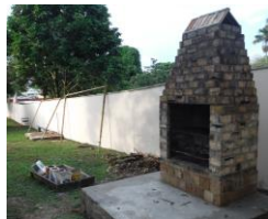
Grill and wash house foundation
